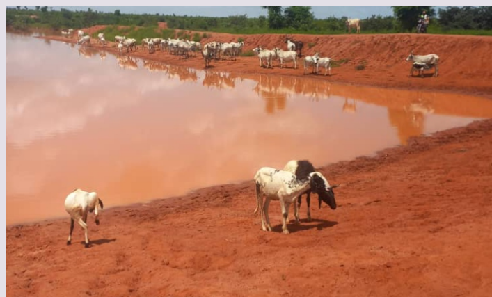
Rain Collection Points (Earth Dam rehabilitated and dredged in Wawa-Zange by Gombe L-PRES Project.
